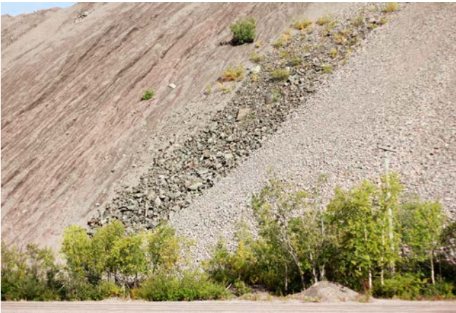
Figure 26. Limited erosion on the WRD outslopes.
